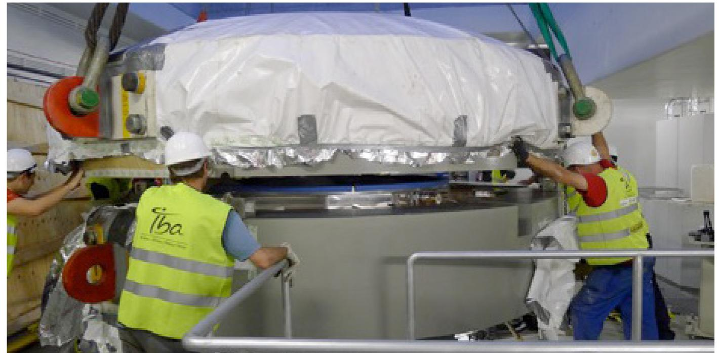
May 11, 2012: Placement of the IBA Proteus 230 MeV proton cyclotron for nuclear research and proton radiotherapy at its site in IFJ PAN in Kraków, Poland.
